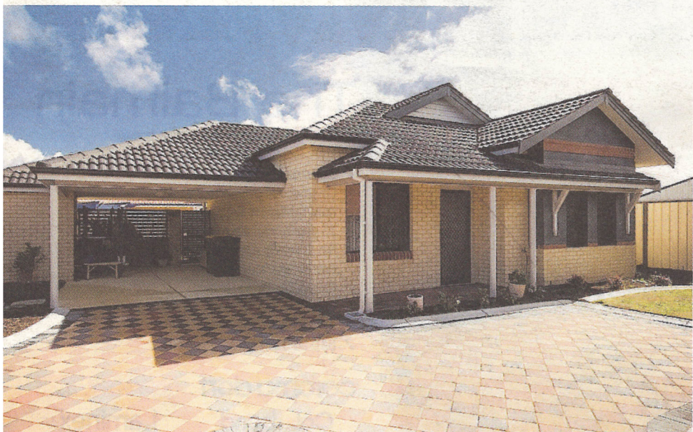
Slim, white-painted poles support verandas across each elevation, shading windows and doors.
